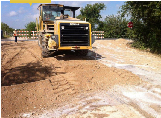
Motor Grader TSW mixing with the soil
