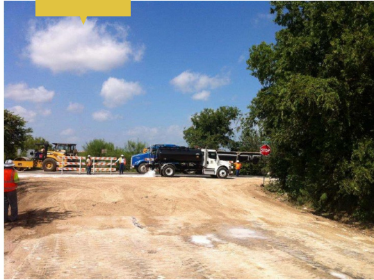
First application of Top-Seal White
