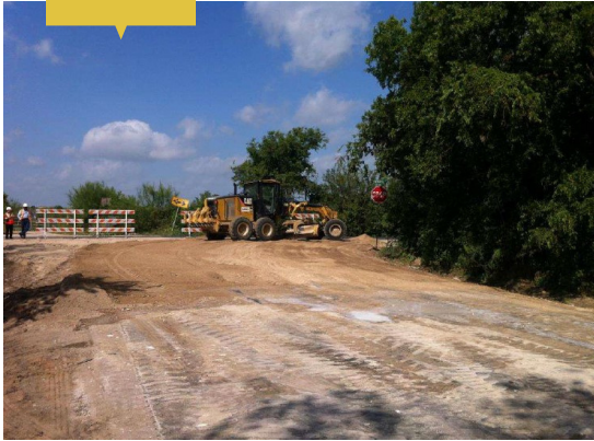
Loose soil prepared for application of TSW
