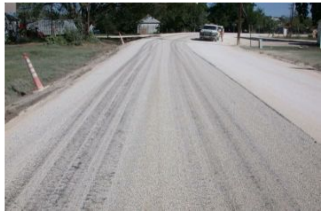
Figure 5- Covered (Inverted) Prime
