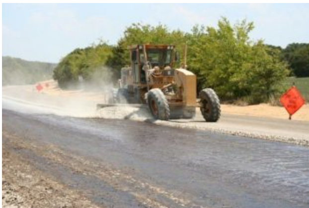
Figure 4- Worked-in (Cut-in) Prime
