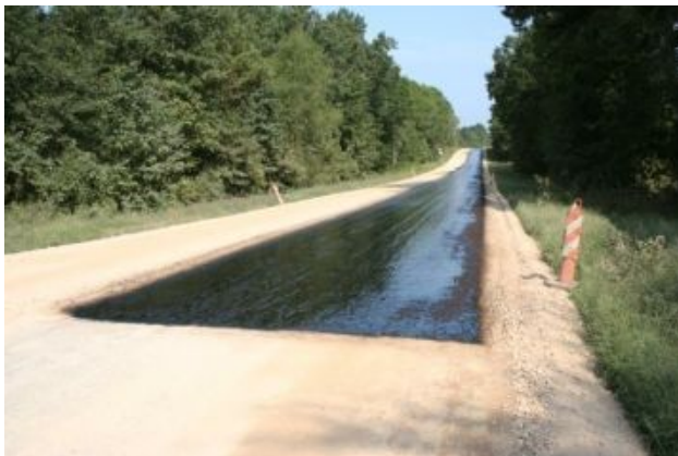
Figure 3- Spray Prime (MC-30, AE-P)
