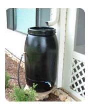
This method is the most common and one that many people are familiar with. This involves installing a barrel at a gutter downspout to collect rainwater. The actual barrel may be a recycled barrel or a new commercially available rain barrel. **Pros:**
