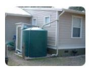
This method is a variation of a rain barrel set-up, but it involves a larger storage volume. Essentially, the collection pipe "drys" after each rain event since it empties directly into the top of the tank. **Pros:**
